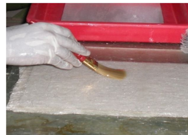
Figure 1 Acetone Cleaning
